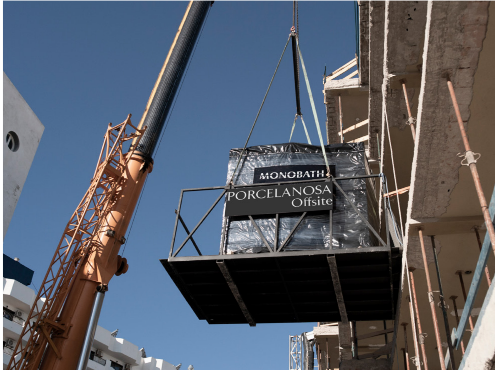
On-site installation prior to placement of façade cladding/walling.
